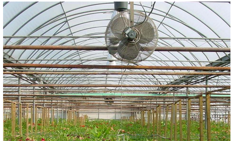
Figure 3. Horizontal airflow fans increase lateral air movement over crops. ( https://bit.ly/2OfntvZ )
