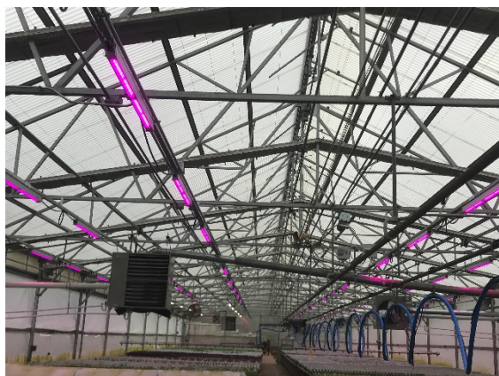
Figure 1. Greenhouse high-pressure sodium (HPS) lamp (above) and light-emitting diode (LED, left) supplemental lighting fixtures.
