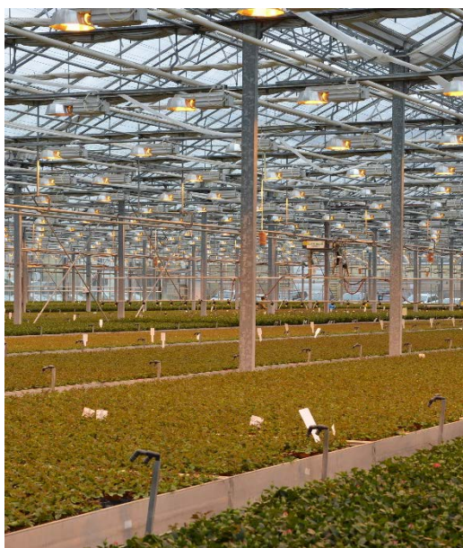
Figure 1. Greenhouse high-pressure sodium (HPS) lamp (above) and light-emitting diode (LED, left) supplemental lighting fixtures.
