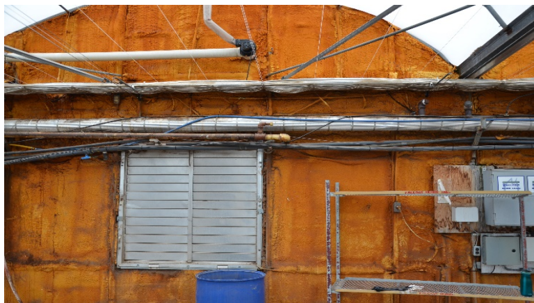
Figure 2. Example of insulating north facing walls with spray foam or insulation board. Photo credit: Roberto Lopez
