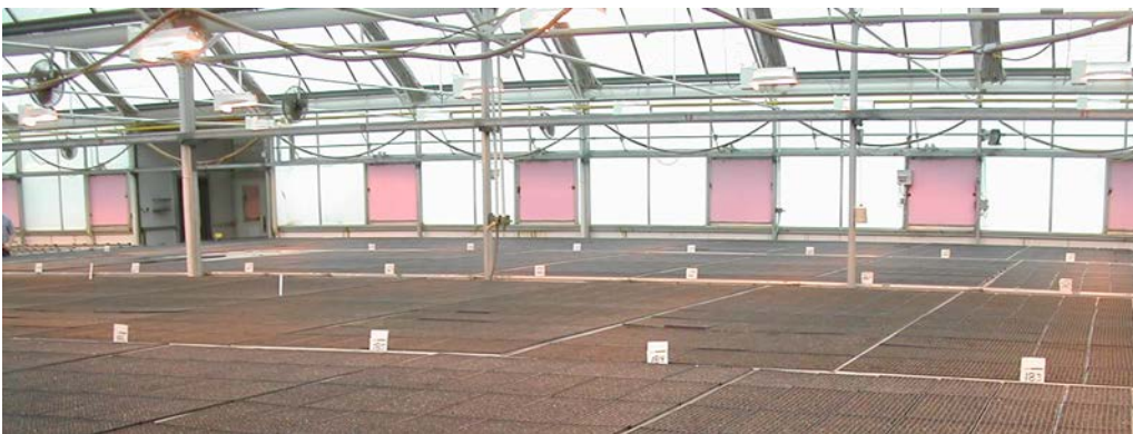
Figure 1. Example of insulating greenhouse end walls or unused exhaust fans with insulation boards. Photo credit: Roberto Lopez
