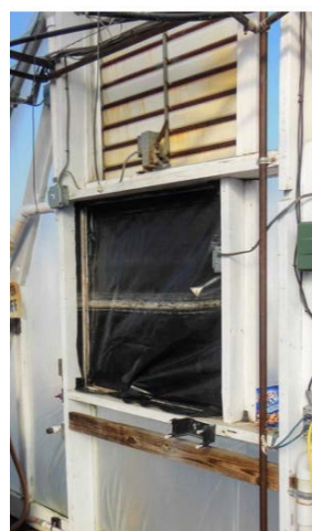
Figure 4. Cover exhaust fan (A) and louver openings (B) inside the greenhouse with plastic, but ensure the fans and/or louvers are off or not in use. Photo credits: W. Garrett Owen and Roberto Lopez
