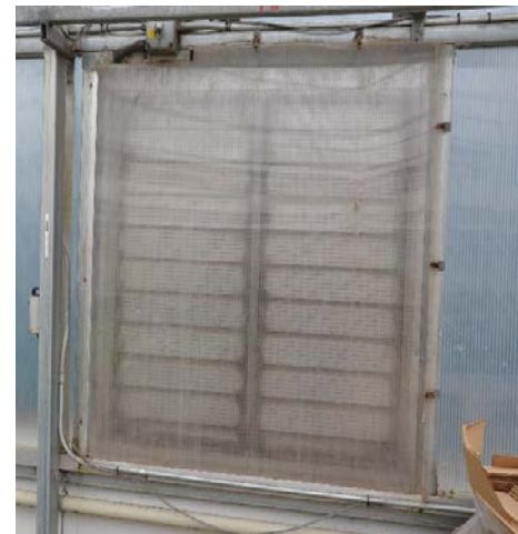
Figure 4. Cover exhaust fan (A) and louver openings (B) inside the greenhouse with plastic, but ensure the fans and/or louvers are off or not in use. Photo credits: W. Garrett Owen and Roberto Lopez
