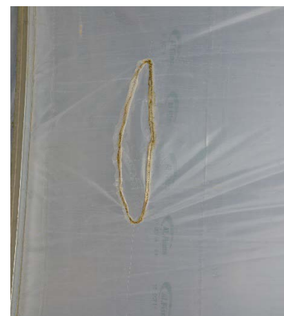
Figure 2. (A) Inspect and repair, (B) patch, and/or replace polycarbonate, acrylic, or other glazing materials that have holes, cracks or tears that may allow heat to escape. Photo credit: Roberto Lopez
