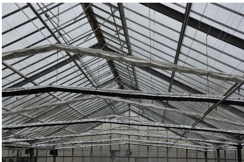
Figure 9. Energy curtains should be deployed to retain heat. Photo credit: W. Roberto Lopez
