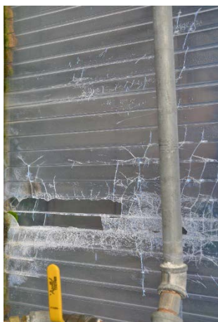
Figure 2. (A) Inspect and repair, (B) patch, and/or replace polycarbonate, acrylic, or other glazing materials that have holes, cracks or tears that may allow heat to escape. Photo credit: Roberto Lopez
